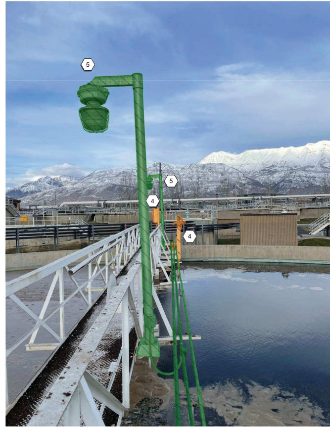
EAST CLARIFIER E-3, VIEW EAST
