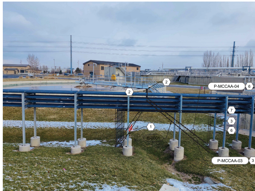
CLARIFIER E-1 CONDUIT RUNS SCALE: NTS
