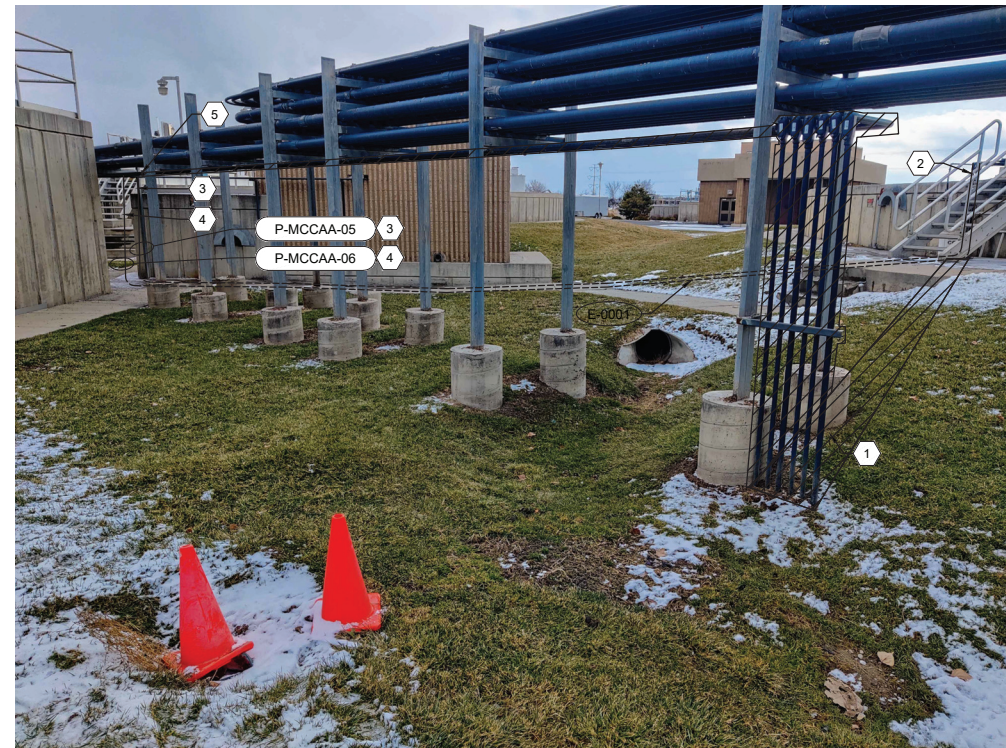
CLARIFIER E-3 CONDUIT RUNS SCALE: NTS
