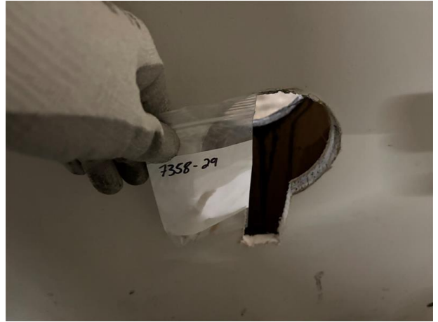
Photo #10 HA-10: Drywall system, not asbestos containing
