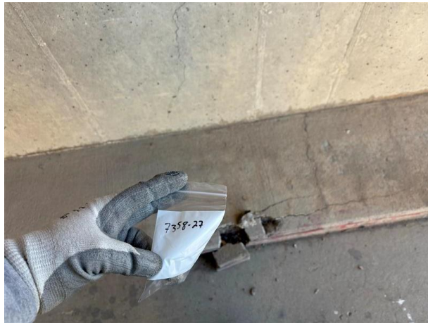
Photo #9 HA-09: Concrete in Loading Dock, not asbestos containing
