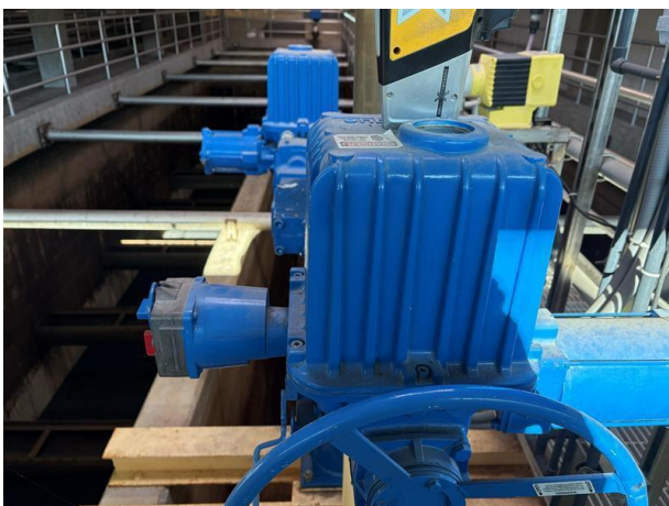
Photo #29 Filter deck blue valve—Lead concentration: 0.26 \text{ mg/cm}^2
