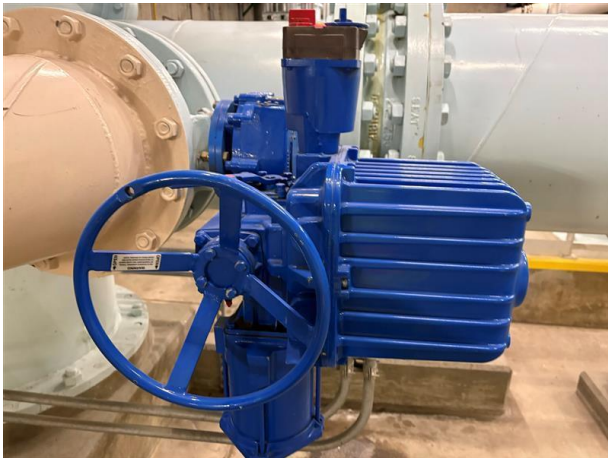
Photo #25 Filter gallery blue valve—Lead concentration 0.04 \text{ mg/cm}^2
