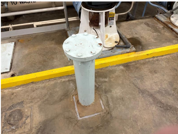
Photo #27 Filter gallery light blue pipe—Lead concentration 0.04 \text{ mg/cm}^2
