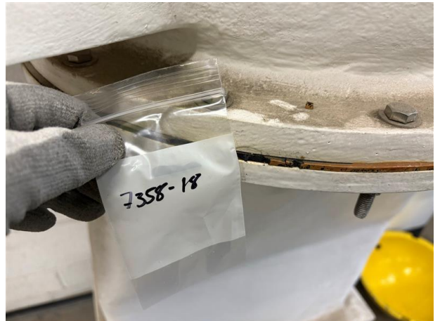
Photo #6 HA-06: Pipe gasket material in Chlorine Room, not asbestos containing
