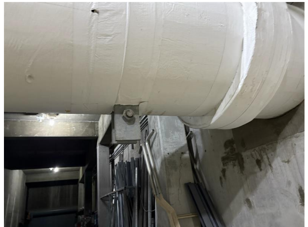
Photo #38 January 31, 2025: Filter gallery new side, gray pipe hanger on north backwash header—Lead concentration: 0.10 mg/cm 2
