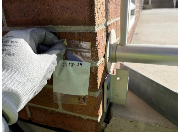
Photo #8 HA-08: Brick and mortar, not asbestos containing
