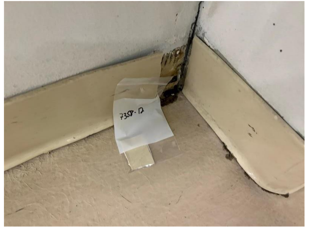
Photo #4 HA-04: Tan cove base and mastic, not asbestos containing
