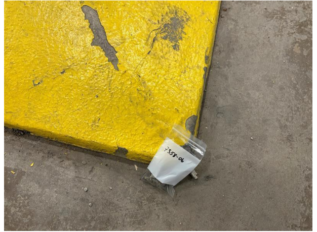
Photo #2 HA-02: Cement in Chlorine Room, not asbestos containing
