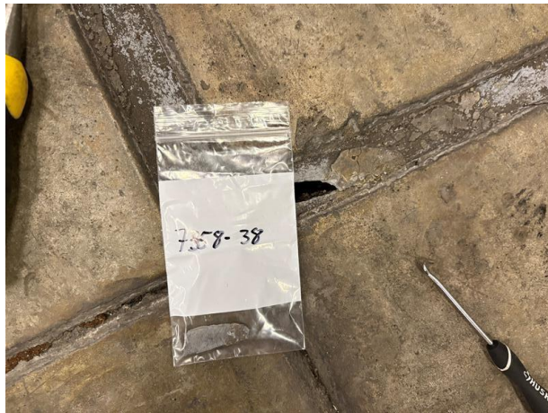
Photo #13 HA-13: Gap filler in basement, not asbestos containing
