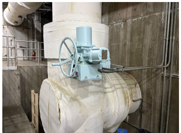
Photo #28 Filter gallery light blue valve—Lead concentration: 0.05 \text{ mg/cm}^2
