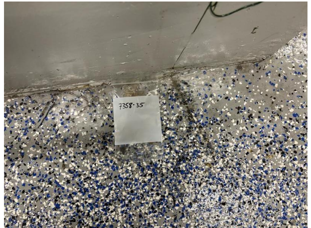
Photo #12 HA-12: Epoxy floor, not asbestos containing
