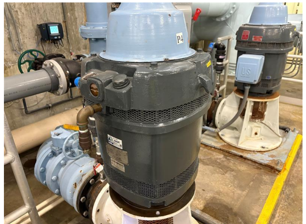
Photo #26 Filter gallery light blue and gray pump—Lead concentration: Light blue 0.04 \text{ mg/cm}^2 , dark gray 0.03 \text{ mg/cm}^2
