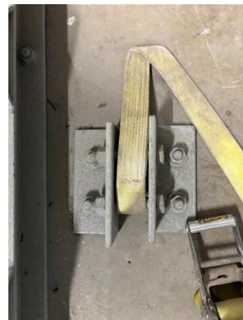
Photo #16 Chlorine storage rack anchor—Lead concentration: 0.10 mg/cm 2
