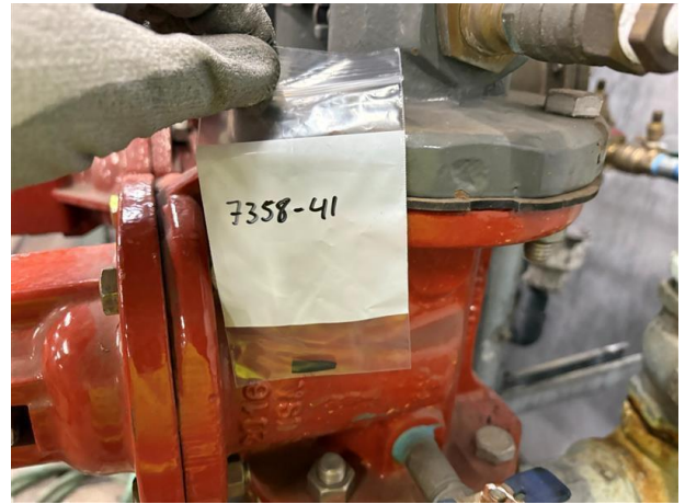
Photo #14 HA-14: Pipe gasket material in basement, not asbestos containing
