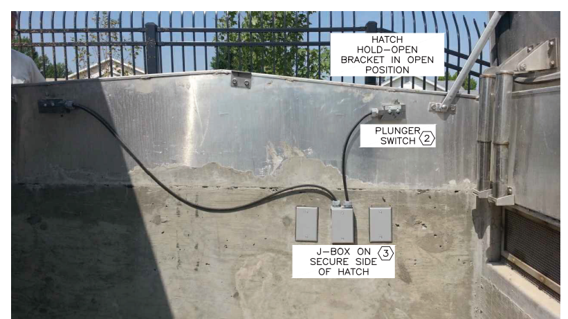
HINGED HATCH SWITCH INSTALLATION 5 3/4" = 1'-0" E5.1
