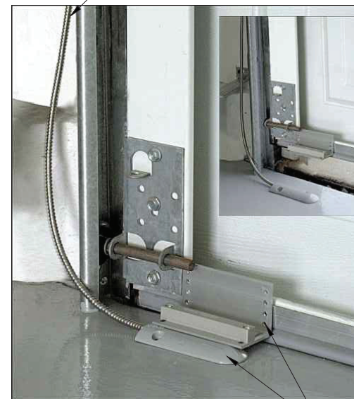
FLOOR MOUNTED SWITCH. MANUFACTURED BY GEORGE RISK INDUSTRIES, INC. MODEL 220-36 OR EQUAL
