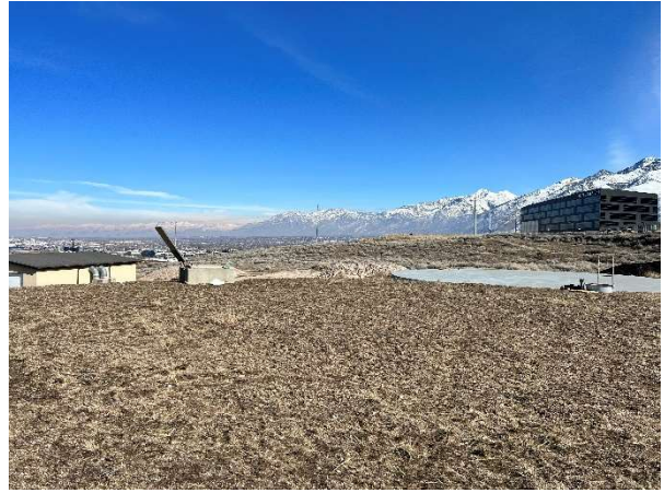
Reservoir roof looking north
