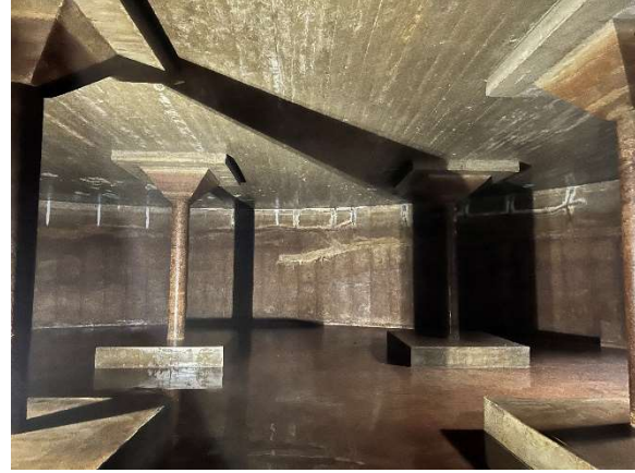
Column connection at roof
