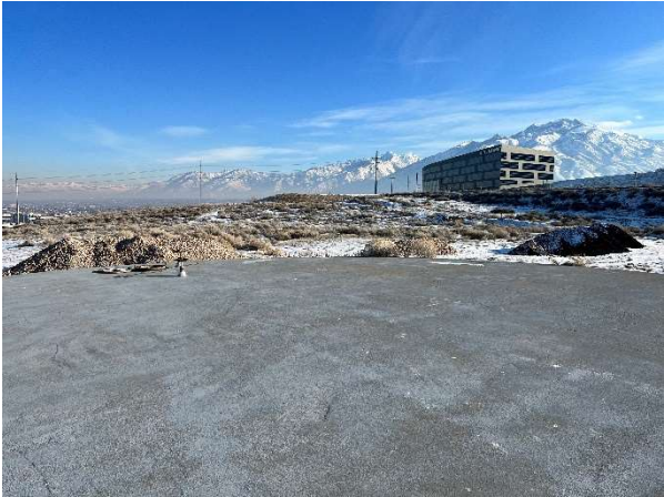
Reservoir roof looking east
