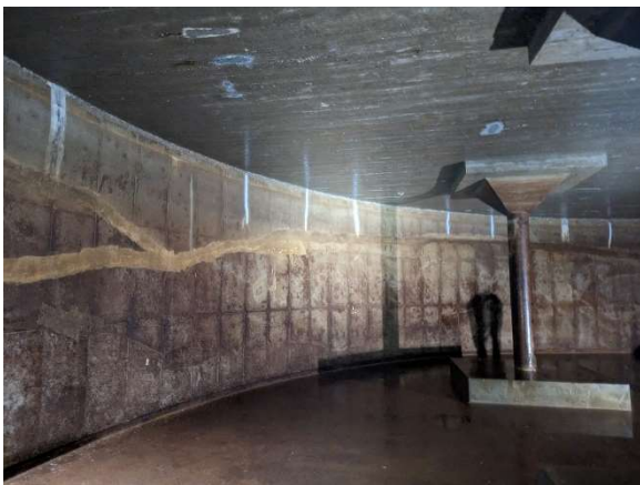
Wall and roof
