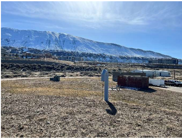
View of reservoir looking south – air vent
