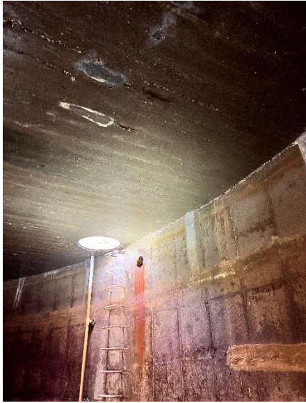
Roof near access manway
