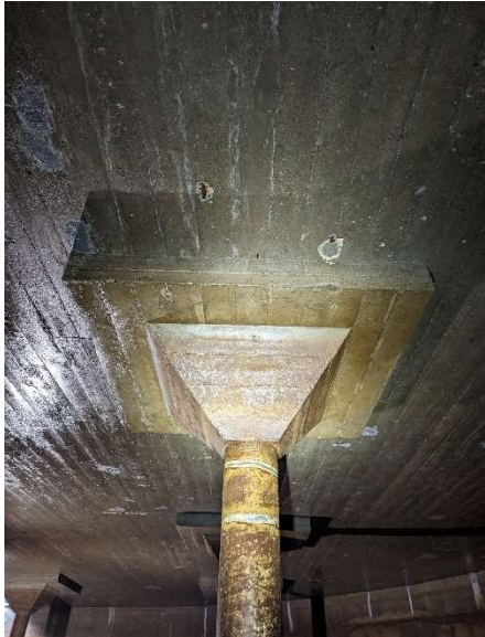
Column drop cap and lid slab
