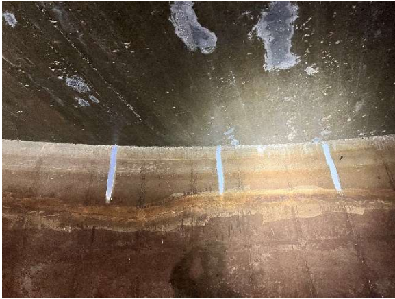
Patched wall cracks at roof joint and slab spall patches
