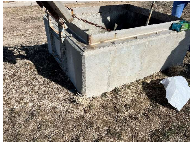
Exterior of the access manway and hatch
