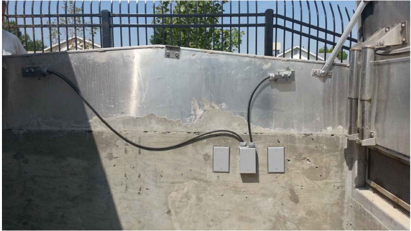
(TYPICAL HATCH INTRUSION SWITCH INSTALLATION)
