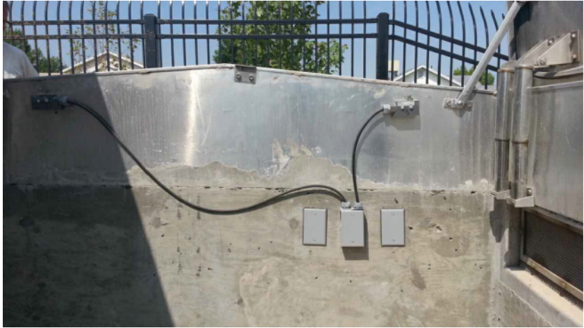
(TYPICAL HATCH INTRUSION SWITCH INSTALLATION)
